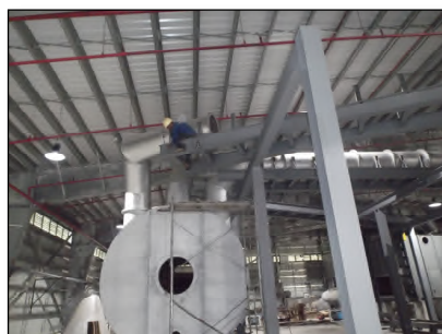
TOPS Gasifiers on foundations (Left) together with Boiler and Secondary Syngas Oxidizer (Right)
