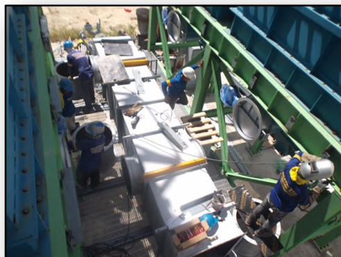
TOPS Gasifiers on foundations (Left) together with Boiler and Secondary Syngas Oxidizer (Right)
