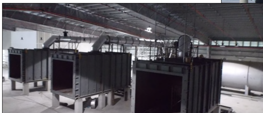
Left: Picture of site taken from Knowles Building (above). Knowles will purchase cold water generated by the TOPS plant using the absorption chillers shown above.
