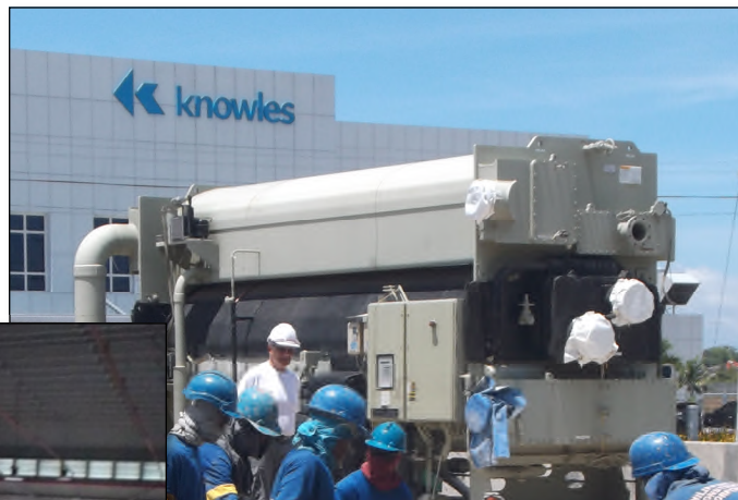
Left: Picture of site taken from Knowles Building (above). Knowles will purchase cold water generated by the TOPS plant using the absorption chillers shown above.
